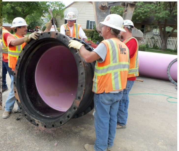
Access Road Preparation at Mid Point of Canyon Segment
