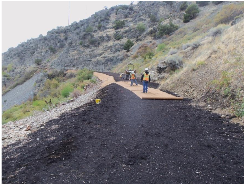
Placed compost in the Canyon Segment
