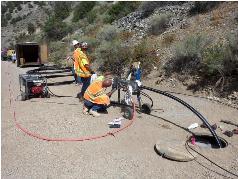
**Installation of the fiber optic cable into the conduit**
