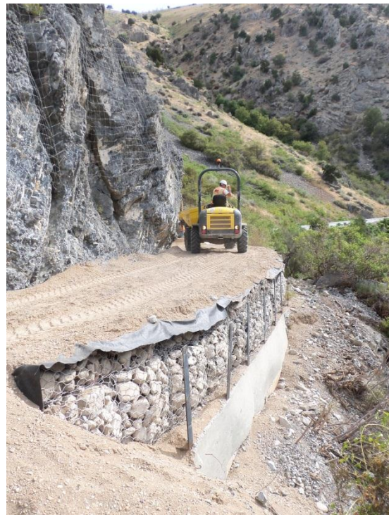
Hauling material over the newly placed gabion wall
