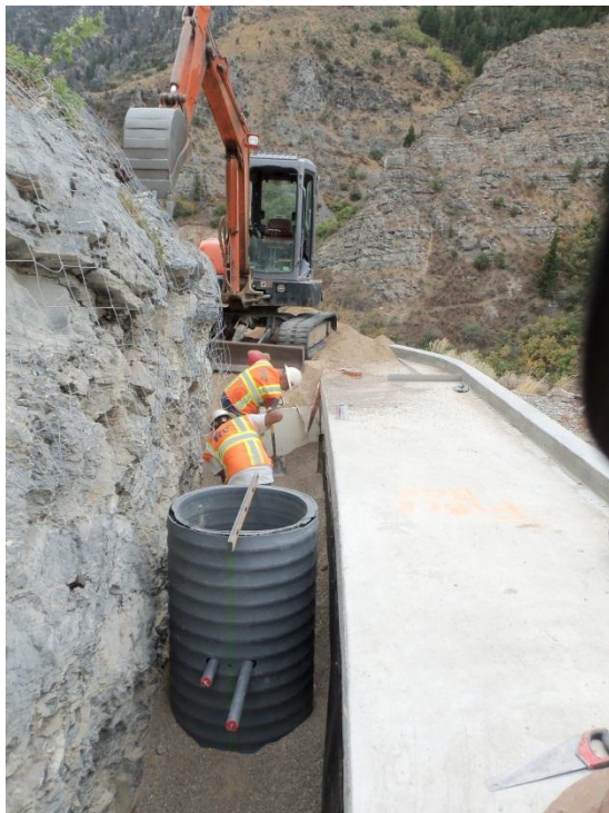
Placement of fiber optic pull box
