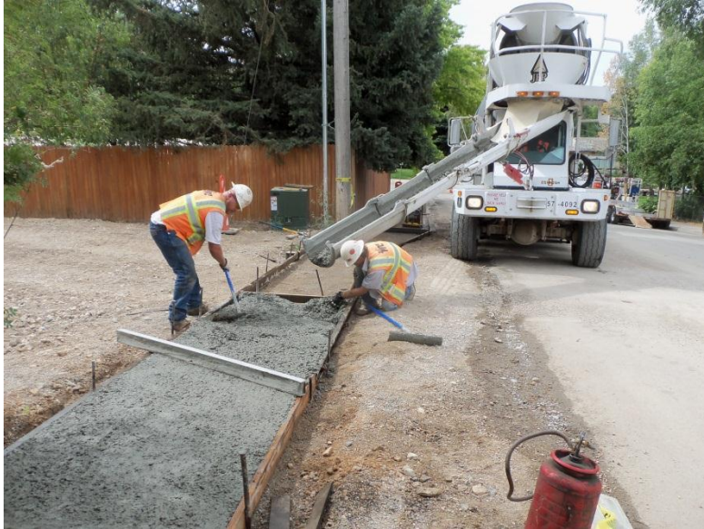
Placement of sidewalk on Cedar Heights Dr.
