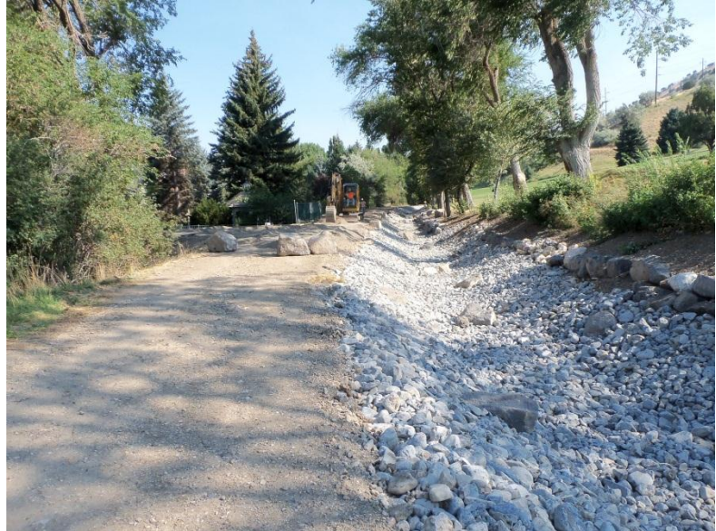
Completed channel near the access road turnaround
