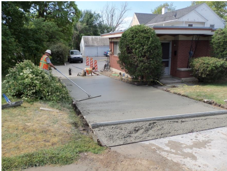
Placement of concrete in the drive way near 600 E and 400 N
