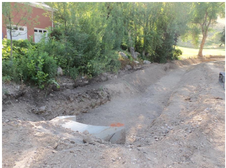
Excavated channel south of Cedar Heights Dr.
