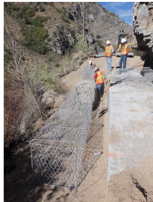
Gabion basket wall below Windy Point
