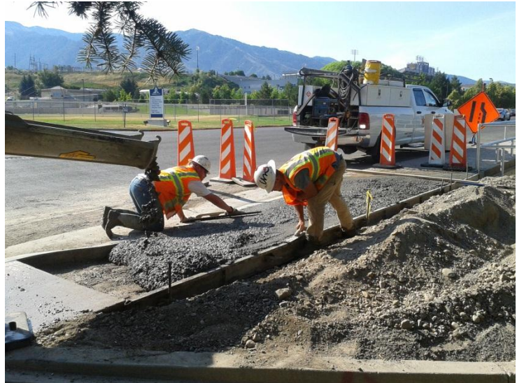
Installation of drive approach on 800 E
