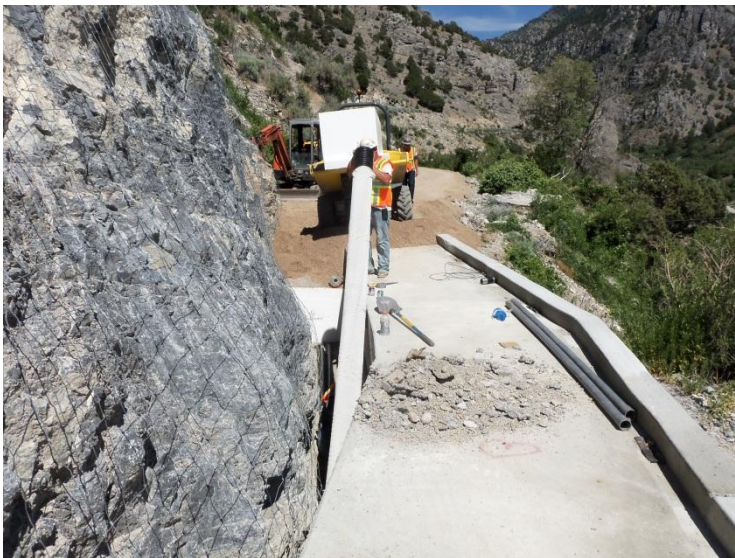
Backfill on box culvert in canyon segment
