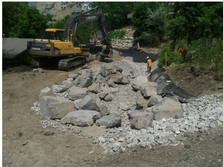
Placement of boulders in landscaped channel
