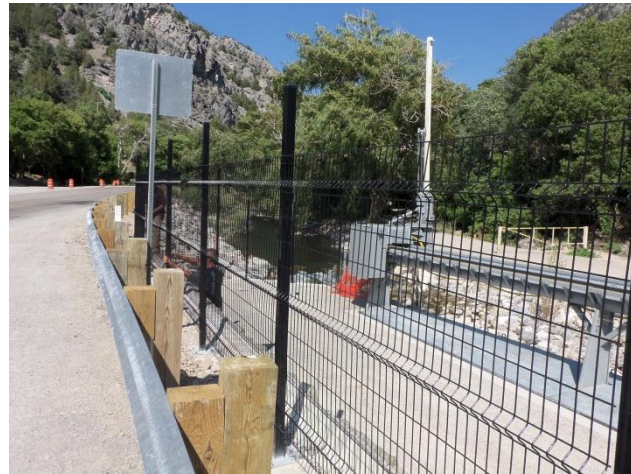
Fencing around the river diversion
