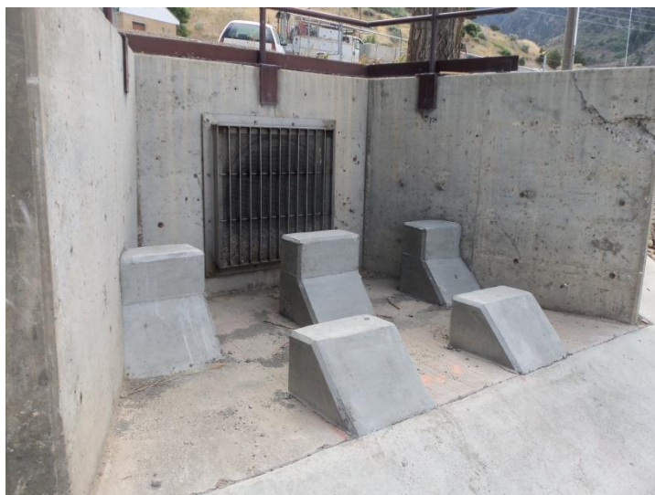
Baffle blocks in front of Logan City tank drain pipe
