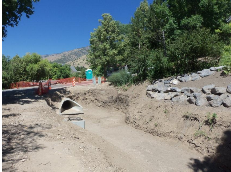
Graded Channel ready for lining near 1220 N
