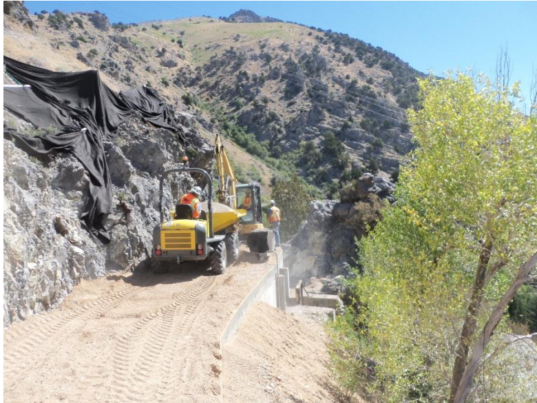
Backfilling box culvert near emergency bypass location
