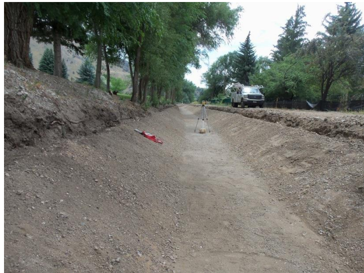
Graded channel ready for lining
