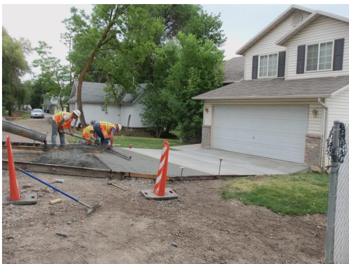
Restoration of driveway disturbed during construction
