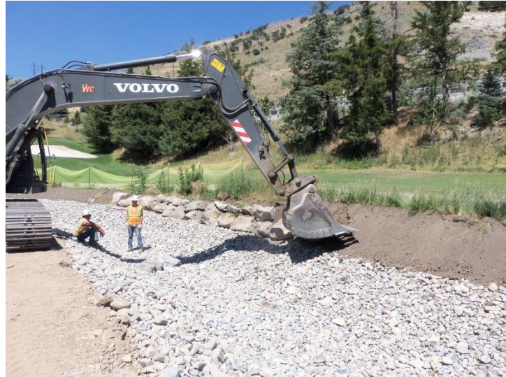
Placement of Rocks to stabilize bank near cart path
