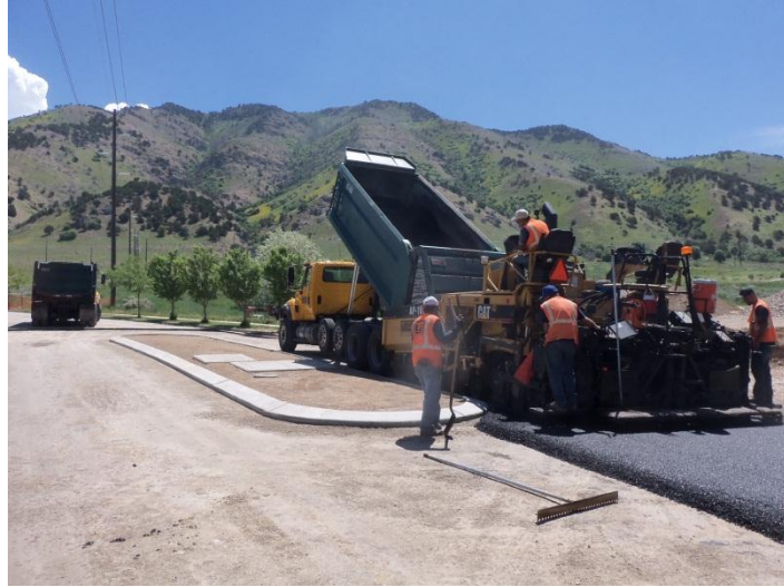
Repaving 1500 N near junction structure
