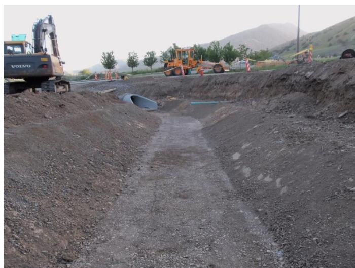
Finished channel ready for lining
