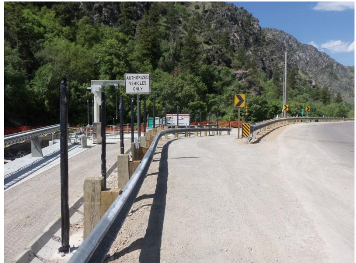
Entrance to diversion structure off of US Highway 89
