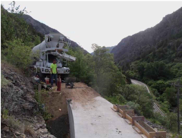
Concrete Truck delivering concrete for curb
