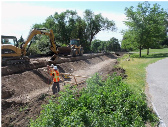
Shaping the landscaped channel inside the Logan Golf and Country Club
