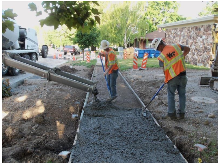
Curb and gutter installation along 600 E
