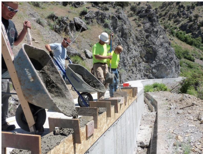
Placement of concrete in curb forms
