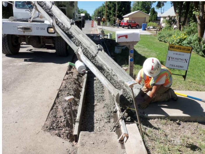
Curb and gutter installation along 600 E
