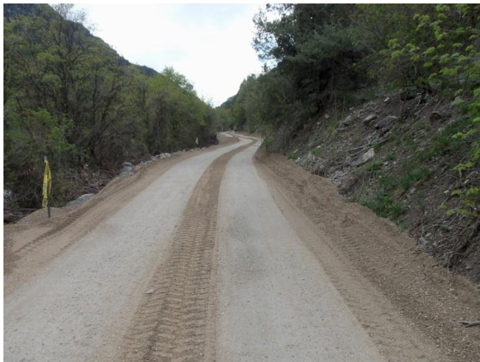
Back fill on the upper section of pre-cast box
