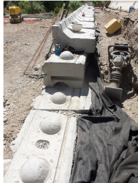
Retaining wall installation
