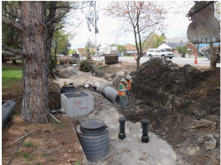
Installation of the storm drain between 400 N and 600 E
