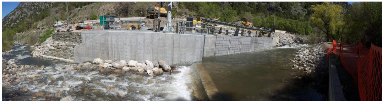
Water running through diversion structure
