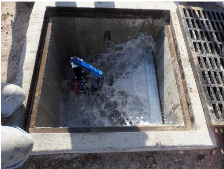
Gravity turnout energy dissipation box
