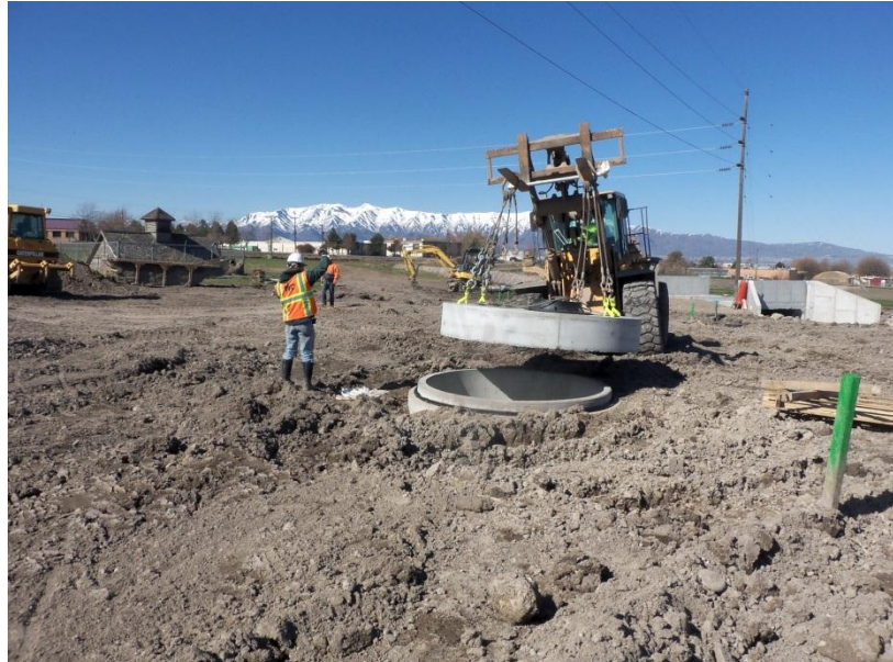
Placing a lid on the 96 inch man hole
