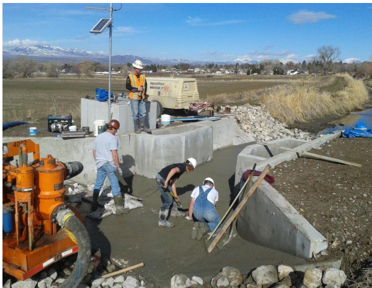
Construction of the Cut Throat Flume at 3100 N
