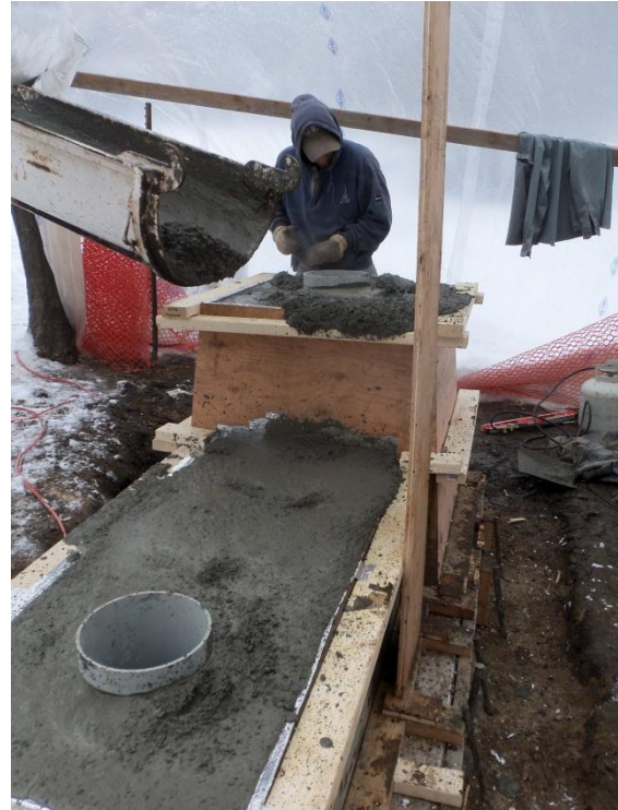
Placement of concrete for the Kiosk base
