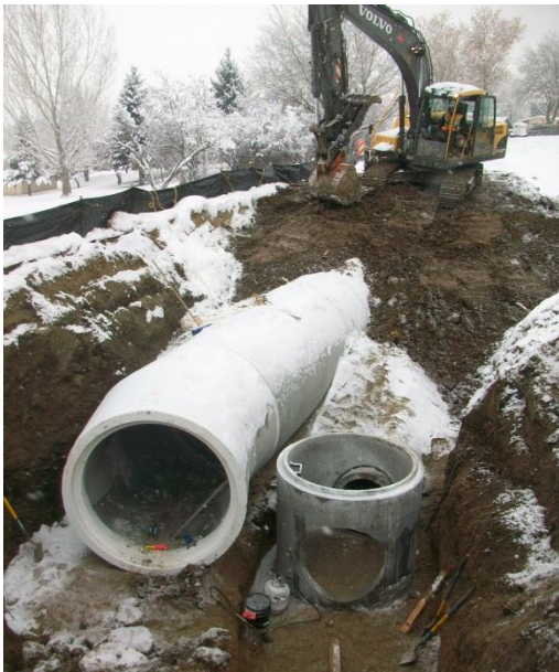
66 inch bend and storm drain manhole placement
