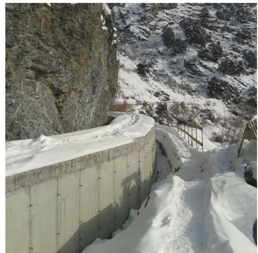
Completed box around a rock face wall
