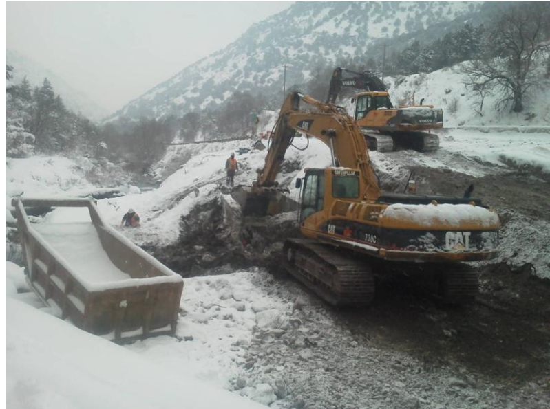
Demolition of existing structure
