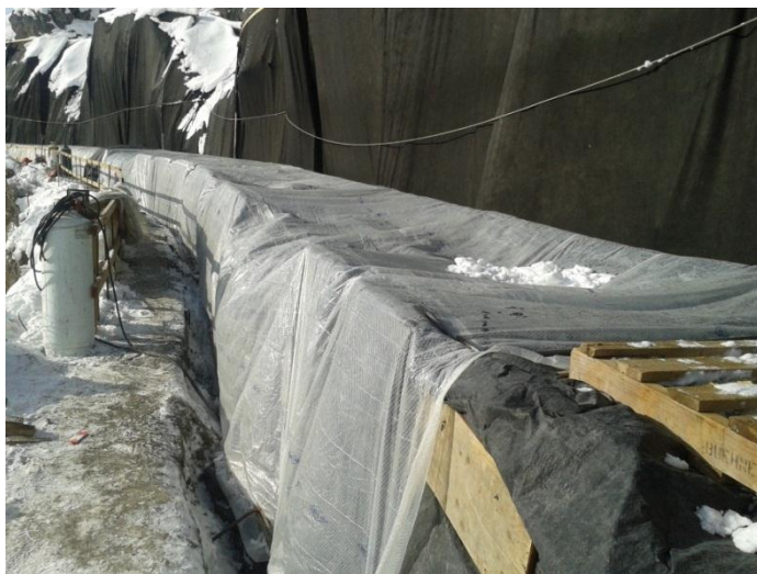
Concrete cold weather protection
