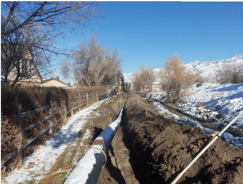
Installing pipe in the existing west canal bank
