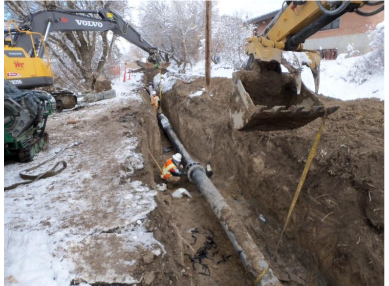
Connection of bored pipe at 1000 N
