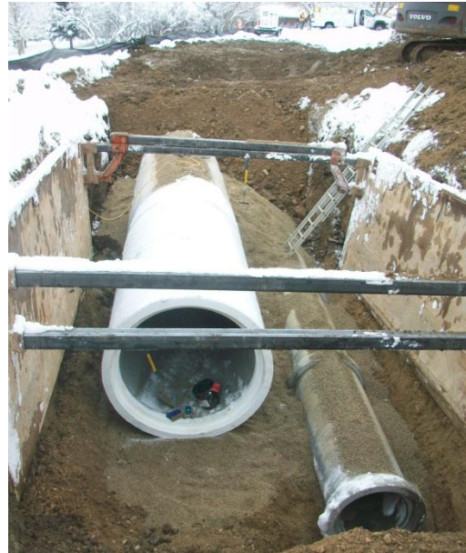
Parallel 66 and 30 inch pipe placement inside trench box
