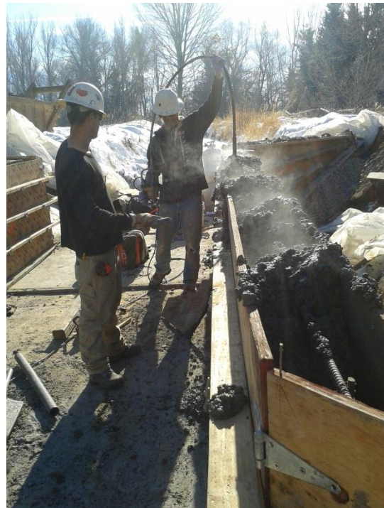
Vibrating concrete in the 3100 N upper flume wall forms
