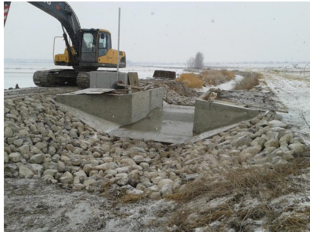
Completion of lower 4400 N flume
