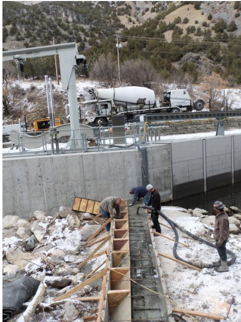
Placement of concrete for the raised sill wall
