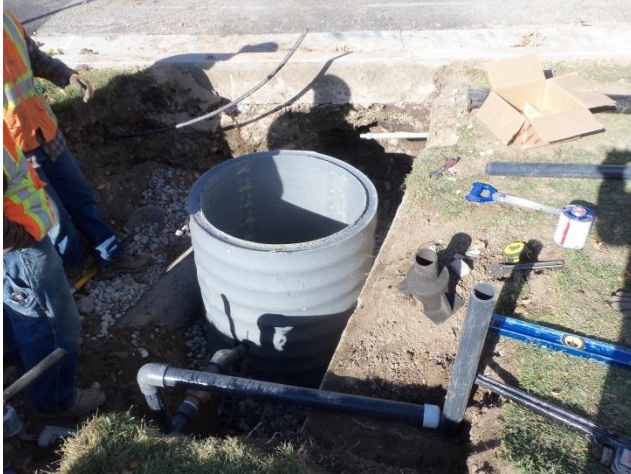
Installation of two inch turnout
