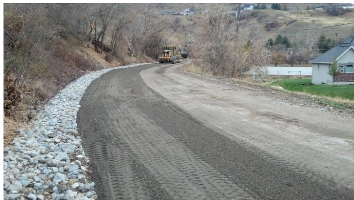
Placement and grading of road base along access road
