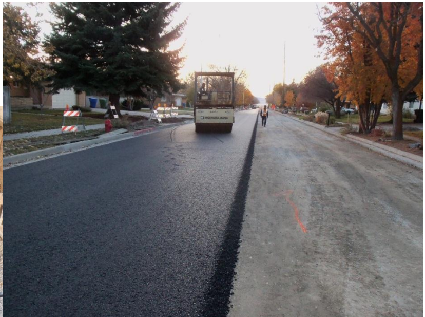
Paving half of the road between 1600 E and 1800 E
