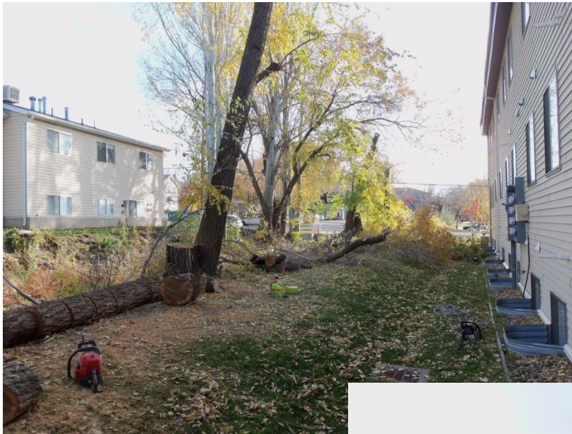
Tree removal near 800N and 600 E on the Logan Northern Segment
