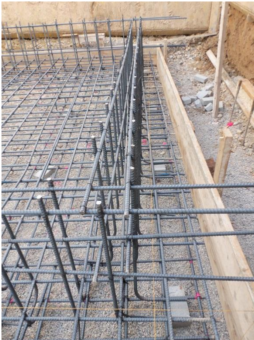
Rebar in the Diversion Structure
