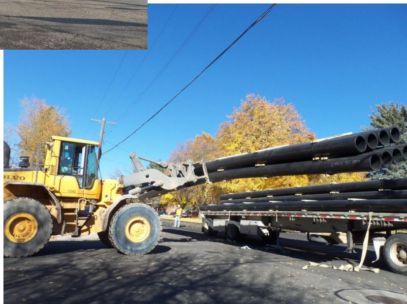
HDPE Pipe Arriving on the Job Site
