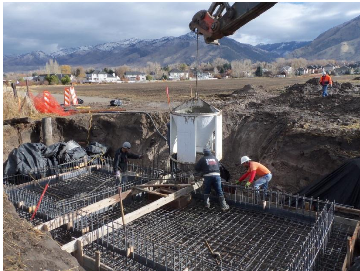
Concrete Placement at the Pressure Reducing Structure
