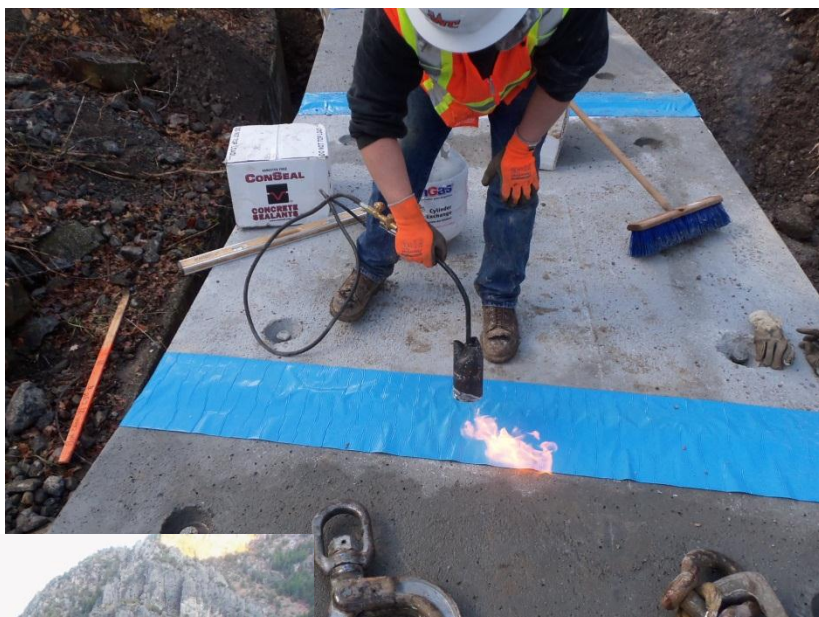
Placing Joint Protection on Precast Section
