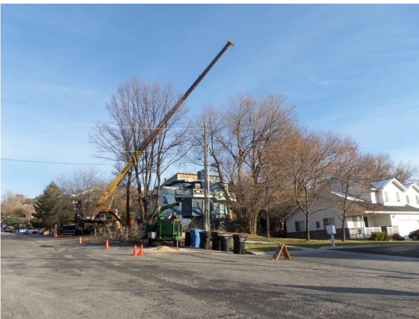
Tree Trimming on the L&N Alignment
