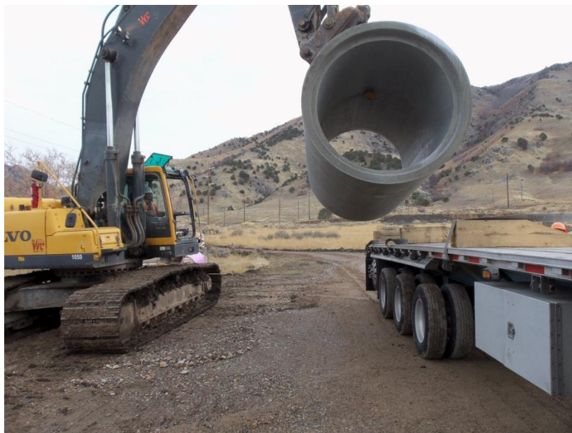
Unloading a 66" RCP from the Truck
