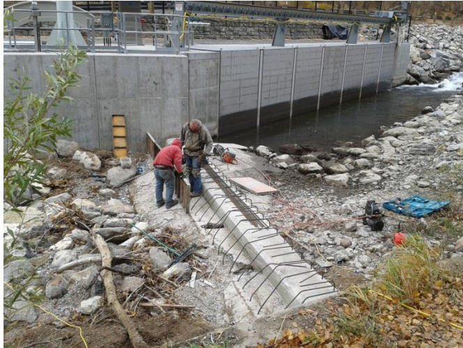
Installing rebar for sill wall adjustment
