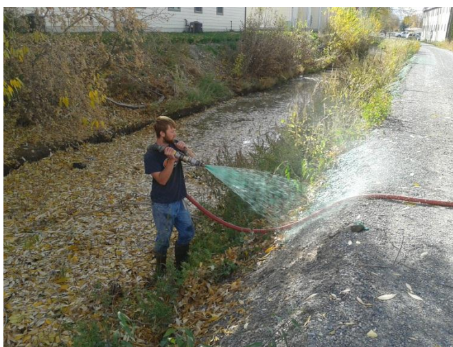
Hydro-seeding a bare portion of canal bank
