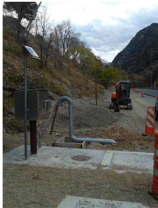
Air vent pipe installed on top of box culvert
