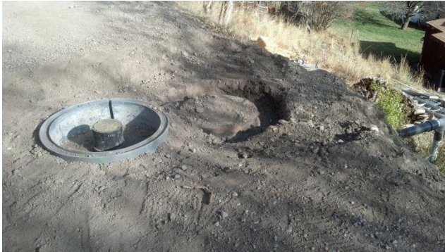
Adjustment of valve box and manhole
