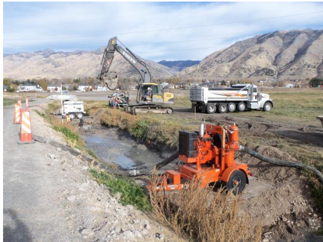
Bi-pass pump diverting water around construction area
