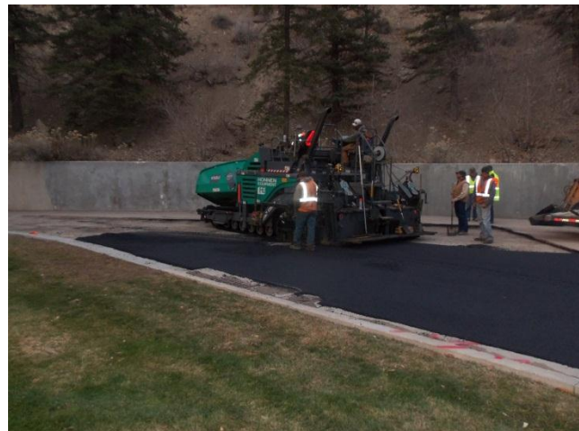
Asphalt placement
