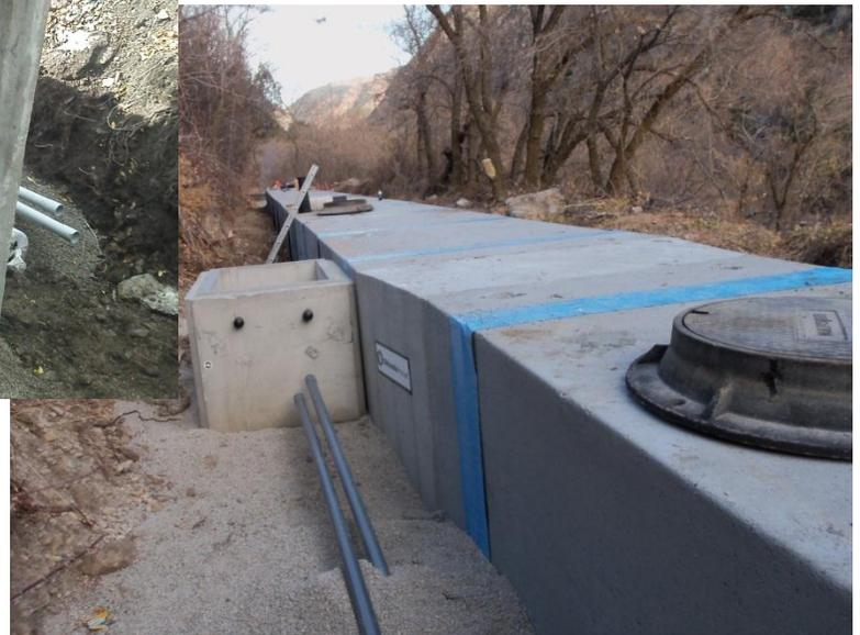
**Cable Pull Box and Box Culvert**
