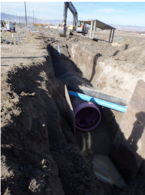
42" pipe under newly placed Drain line and pressure irrigation line in USU Easement
