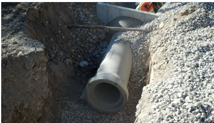
Placement of concrete pipe across Ropes Course Road
