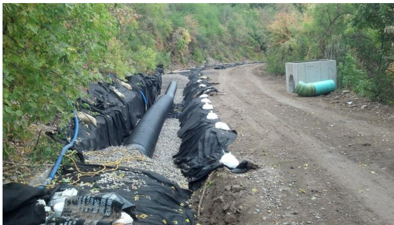
East Turn out box with cut off wall
