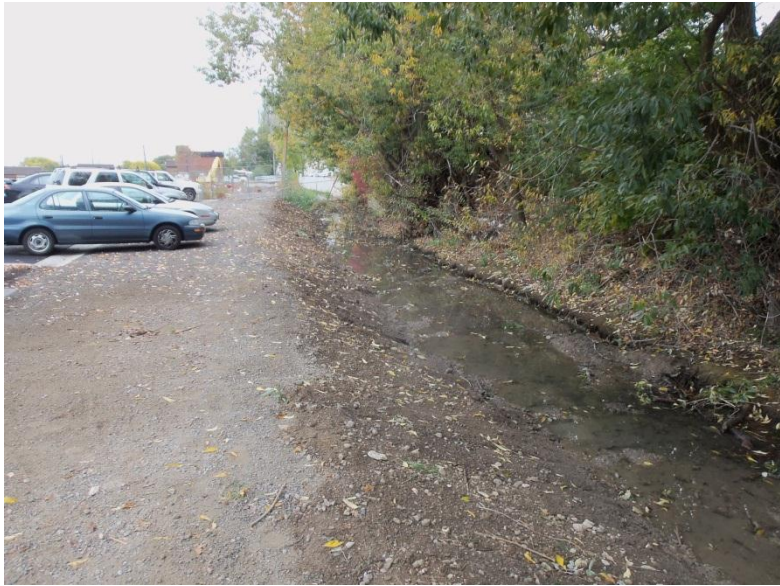
Reshaping of canal bank to specified slope
