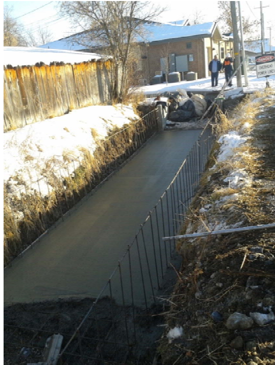
Concrete placement for the slab portion of the concrete lined canal
