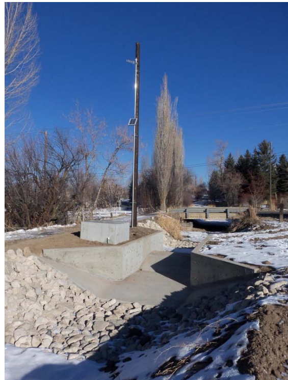
Completed ramp flume on the LHPs Canal near 3100 N
