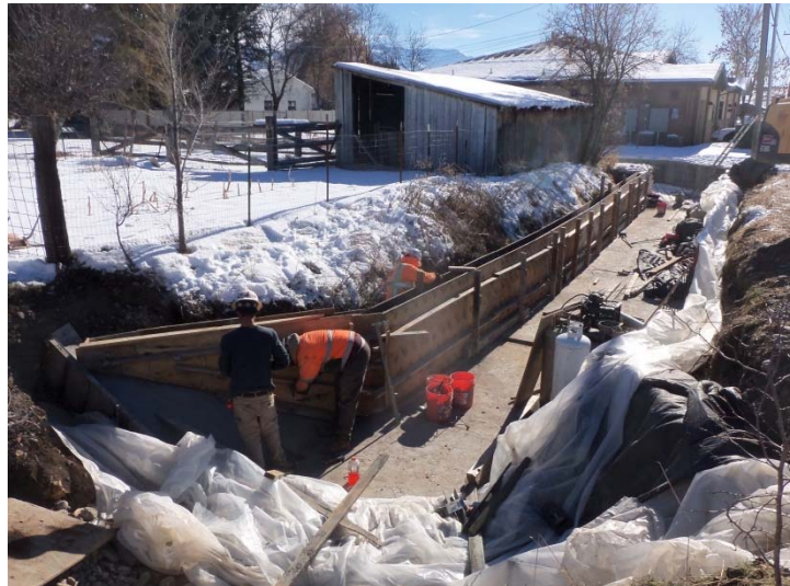
Forming of the east wall of the Smithfield flume
